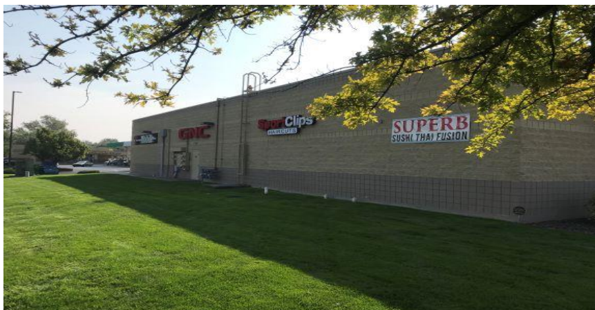
Back of the building facing Greenhurst/12 th Ave intersection
